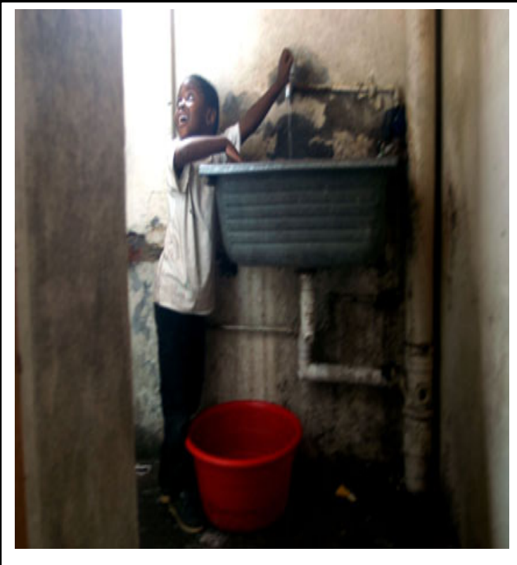
CROWN BUILDING, Carlisle Street, Durban Photograph, Courtesy of KwaZulu Natal Independent Newspapers
